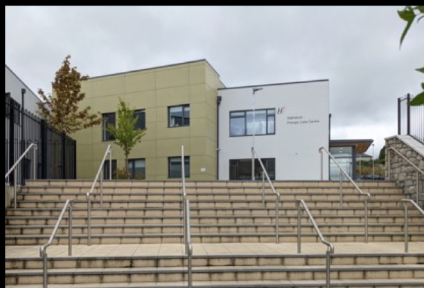
Stairs to door
